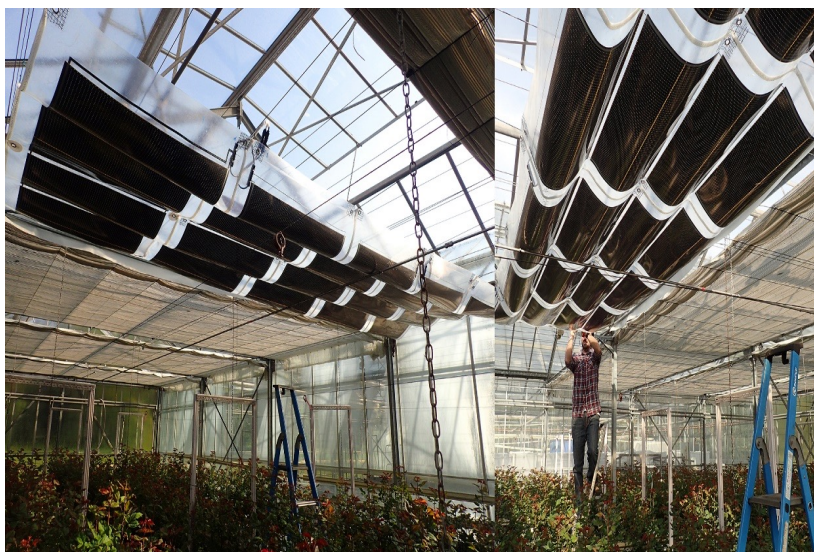
Semi-transparent photovoltaic film easy to roll in/out
